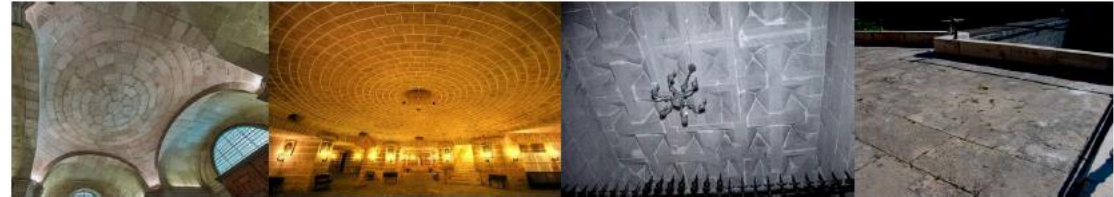
Figure 1: Interlocked vaults examples (from left to right): Monastery of Escorial (1565), Cádiz Cathedral's Crypt (1730), Lugo's Cathedral (1699), Pontón de la Oliva (1853)
